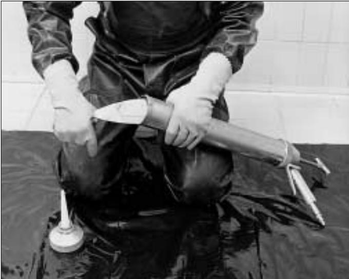
11. The movement jointing compound should be applied with a mastic gun or pointing trowel. A spatula should be used to fill the mastic gun with compound after it has been mixed.
