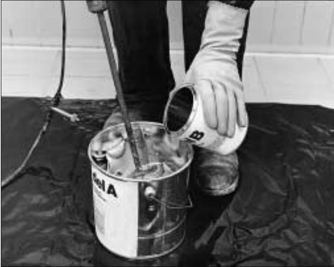
10. When the jointing compound has been applied and allowed to dry, the cellular plastic (see Fig. 9) should be scraped out of the movement joints down to the level of the bottom of the tiles. Check that the edges of the tiles are free of mortar, etc. For optimum adhesion to ceramic, concrete etc. edges of movement joints should be primed with CC Höganäs Primer 37. The movement joints should be filled with CC Höganäs Habenit 50 jointing compound, according to the instructions on the package.
