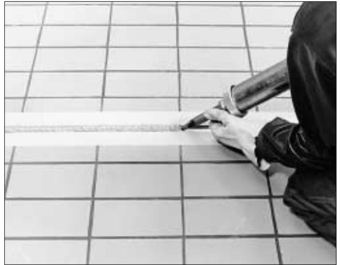
12. Mask either side of the joint with tape before commencing. Prime the movement joint edges with CC Höganäs Primer 37. Fill the movement joint liberally.
