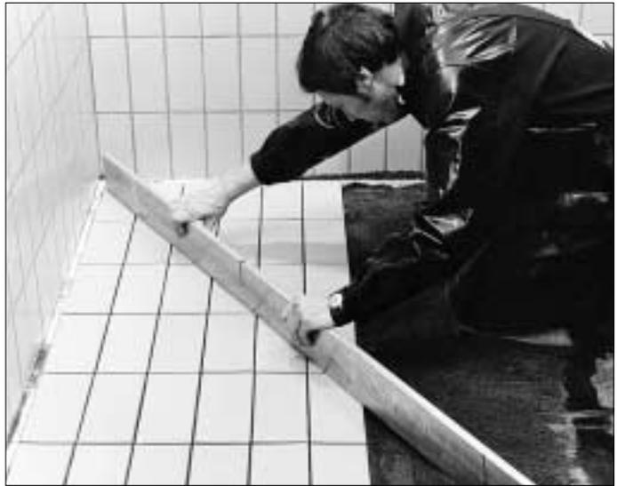
8. The evenness of the surface of each newly laid section should be carefully checked with a gauge float and adjusted if necessary.
