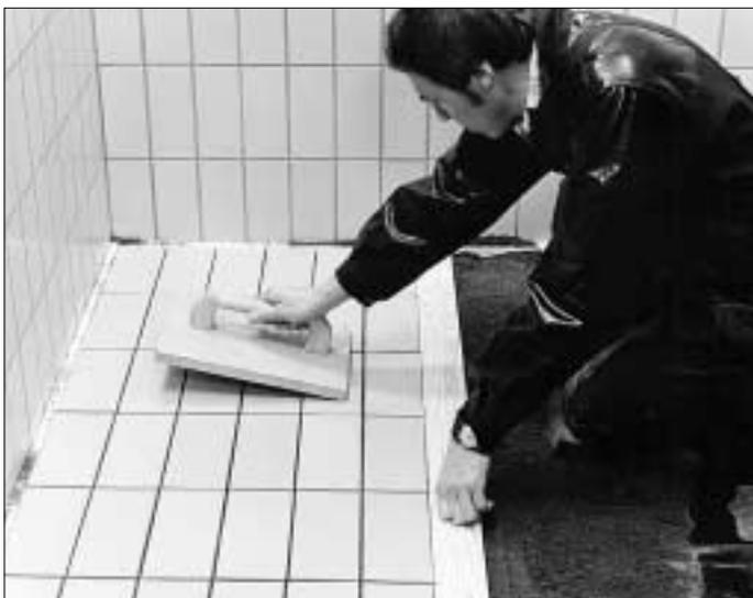
7. The tiles should be tamped down into the slurry.
