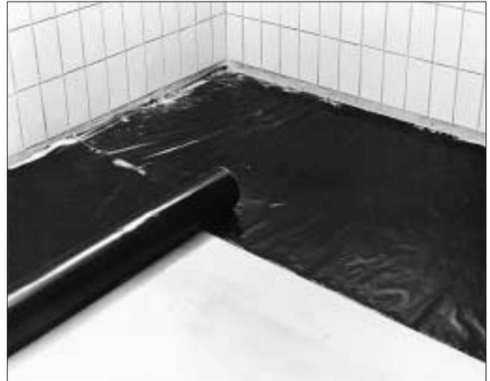
2. A 0.1 mm plastic sheet should be unrolled on the sub-floor. A soft brush should be used to smooth out the sheet and remove any air bubbles. Roll out each sheet so that it overlaps the preceding one.
