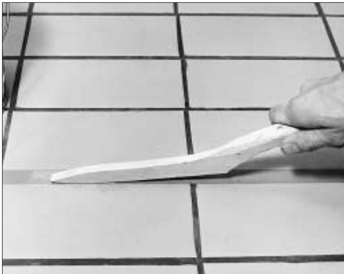
15. After the surface has been allowed to cure for a few minutes, the joint can be smoothed with a flat wooden stick dipped in acetone.
