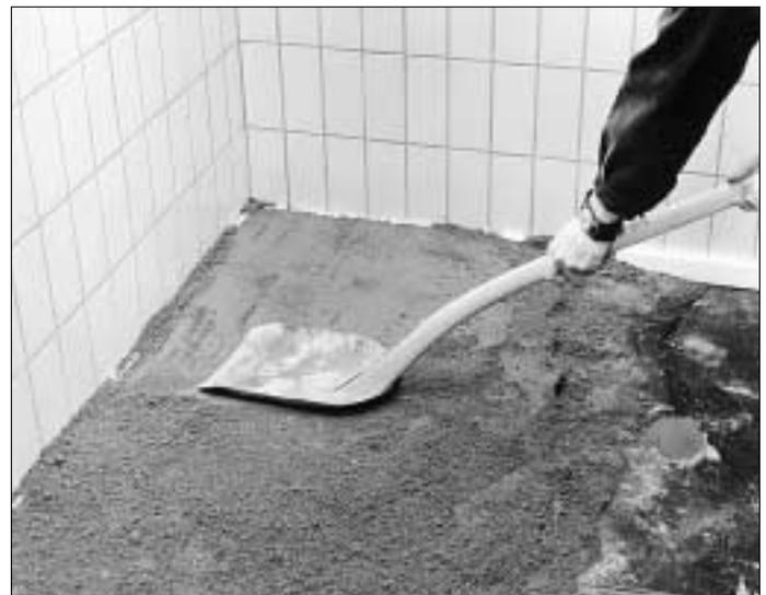
3. Spread out the mortar and compact it carefully. Do not spread out more mortar than is needed for 4–5 courses of tiles at one time.
