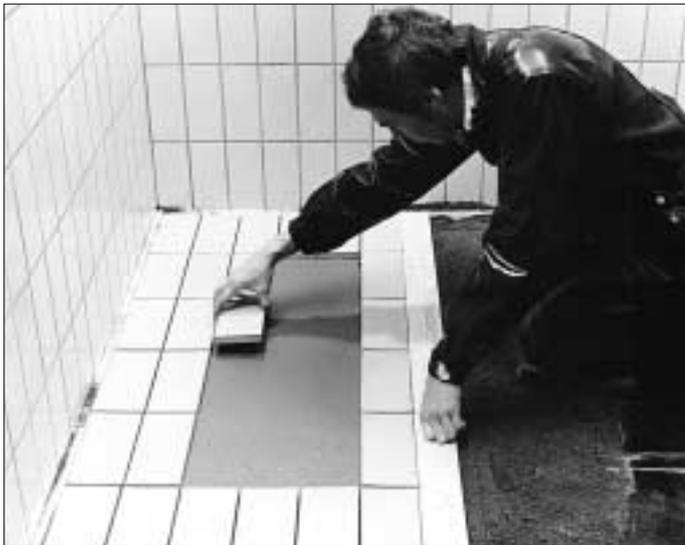
6. When the surplus water has been absorbed by the mortar and the slurry has taken on a matt appearance, the tiles should be laid out according to the markings on the gauge float.
