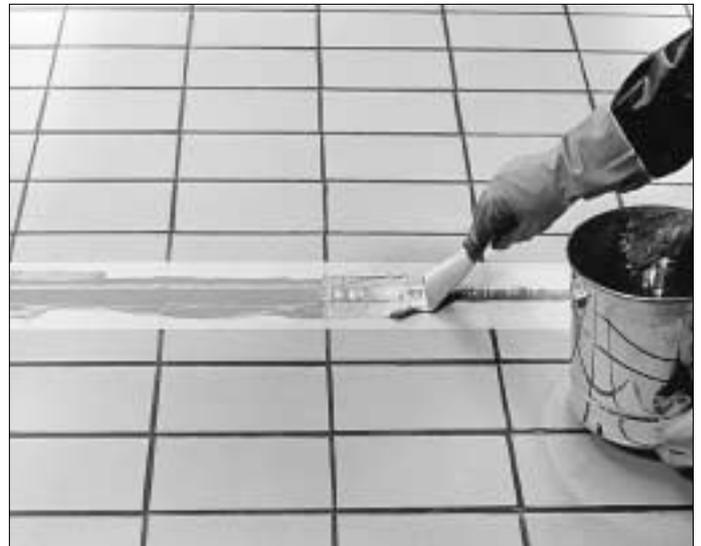
13. Cut away the excess compound, which can be used again, and smooth the surface with a flatbladed palette knife.
