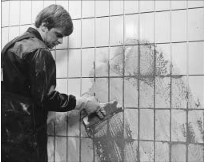
4. The joints between the tiles can be grouted 1 - 2 days after the tiles have been laid. The joints should be free of adhesive to at least half the thickness of the tile. Highly absorbent tiles should be moistened before grouting. Apply the grout diagonally over the joints with a rubber spreader until they are completely filled. Remove excess grout by scraping it off with a spreader.
