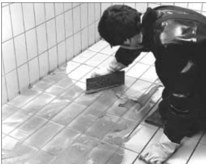
2. Excess grout should be removed with the spatula held at a right angle to the surface and drawn diagonally across the tiles.
