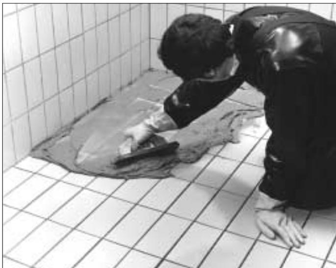
1. A rubber spatula is used to apply the grout, it should be held at an angle to the surface. The grout should be worked down into the joints until they are well filled. Note carefully whether mortar sinks below the tile surface level after application. The grout should be applied along the joints in both directions, so that a wave of grout is formed in front of the spatula.
