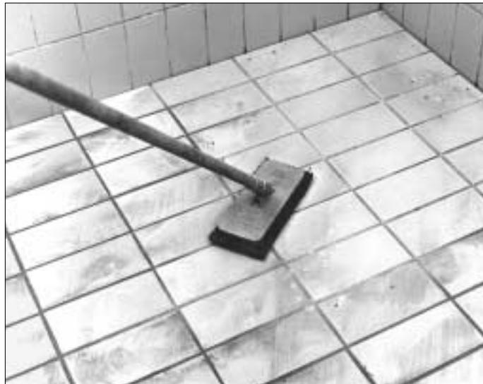
3. Clean the surface 1–2 hours after grouting with water and CC Höganäs scotchbrite FB 93 (on a long holder).
